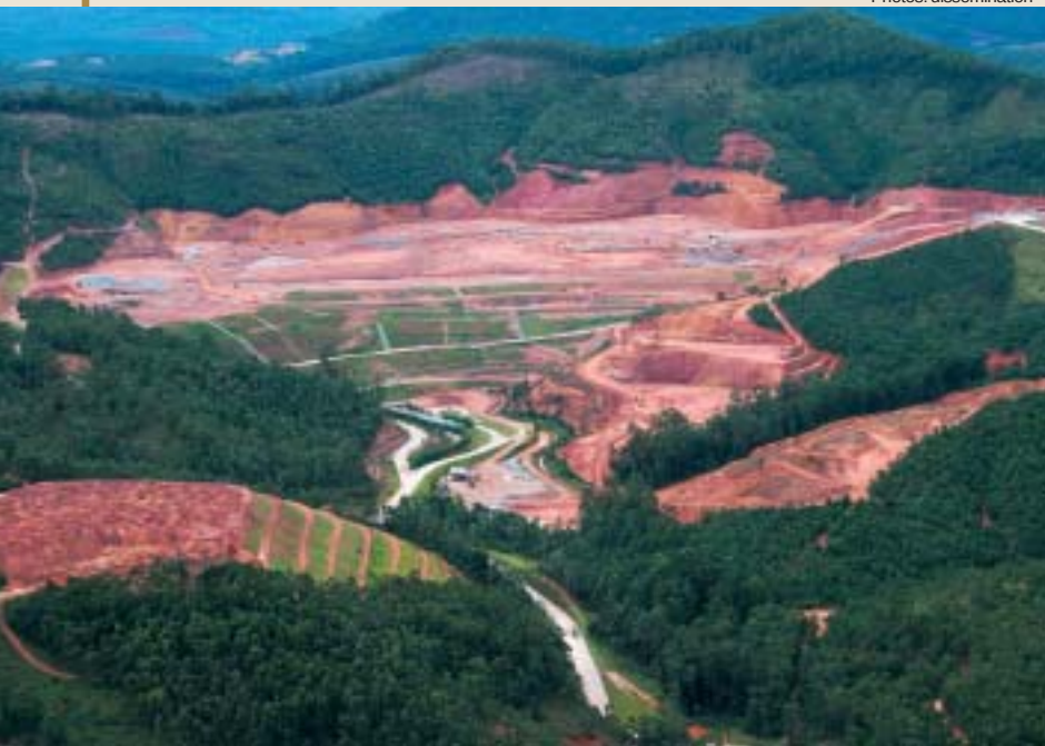
Caieiras CTR: air view
