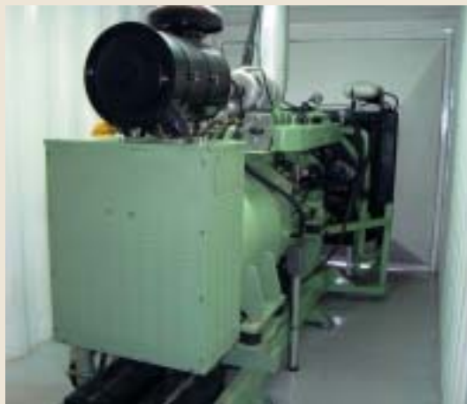
Otto cycle engine, 200 kW power, Brazilian technology
